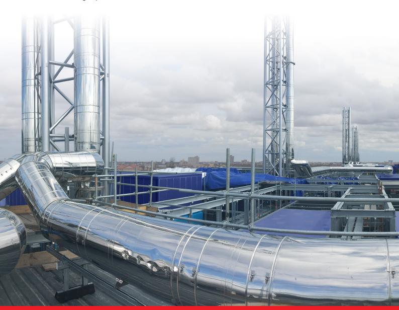
Chimney solutions designed for standby and prime-powered Data Centre diesel and gas generators
